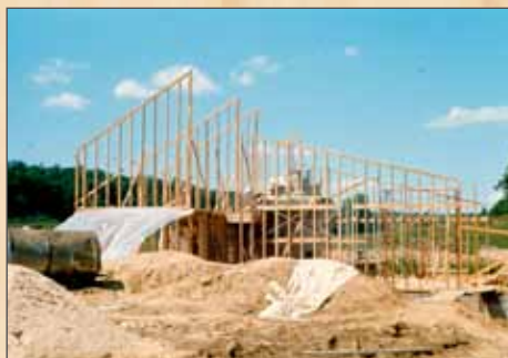
Nature Center under construction (1972)
